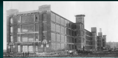
Ford Highland Park Plant, Building A under construction, 1909
