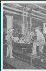
Lowering Motor to Place on Chassis Looking to southeast, shows overhead chain-hold rails
